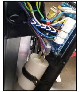
6. Cut the Pump Cable, cable ties, and wind the insulation off the lower loom bulkhead fitting. Loosen the lower bulkhead fitting nut and pull the old cable through the lower bulkhead fitting from the control panel side.
